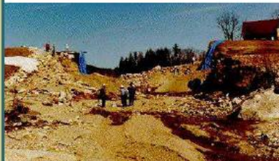
Alton dam breach, 1996
